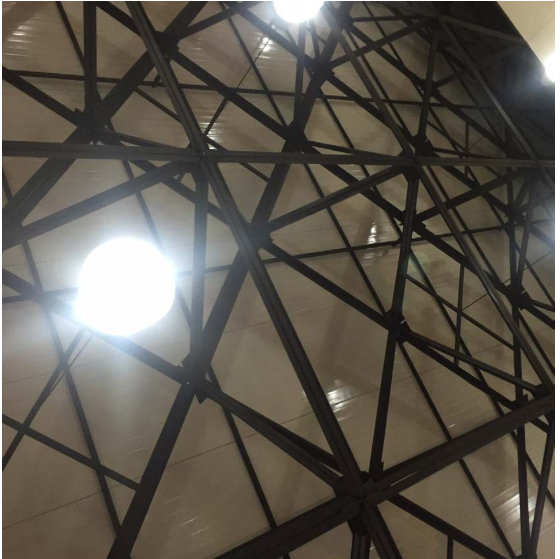
Realizim I mbuleses me panel sandwich per showroom OPEL NOSHI(Dita e inagurimit)
