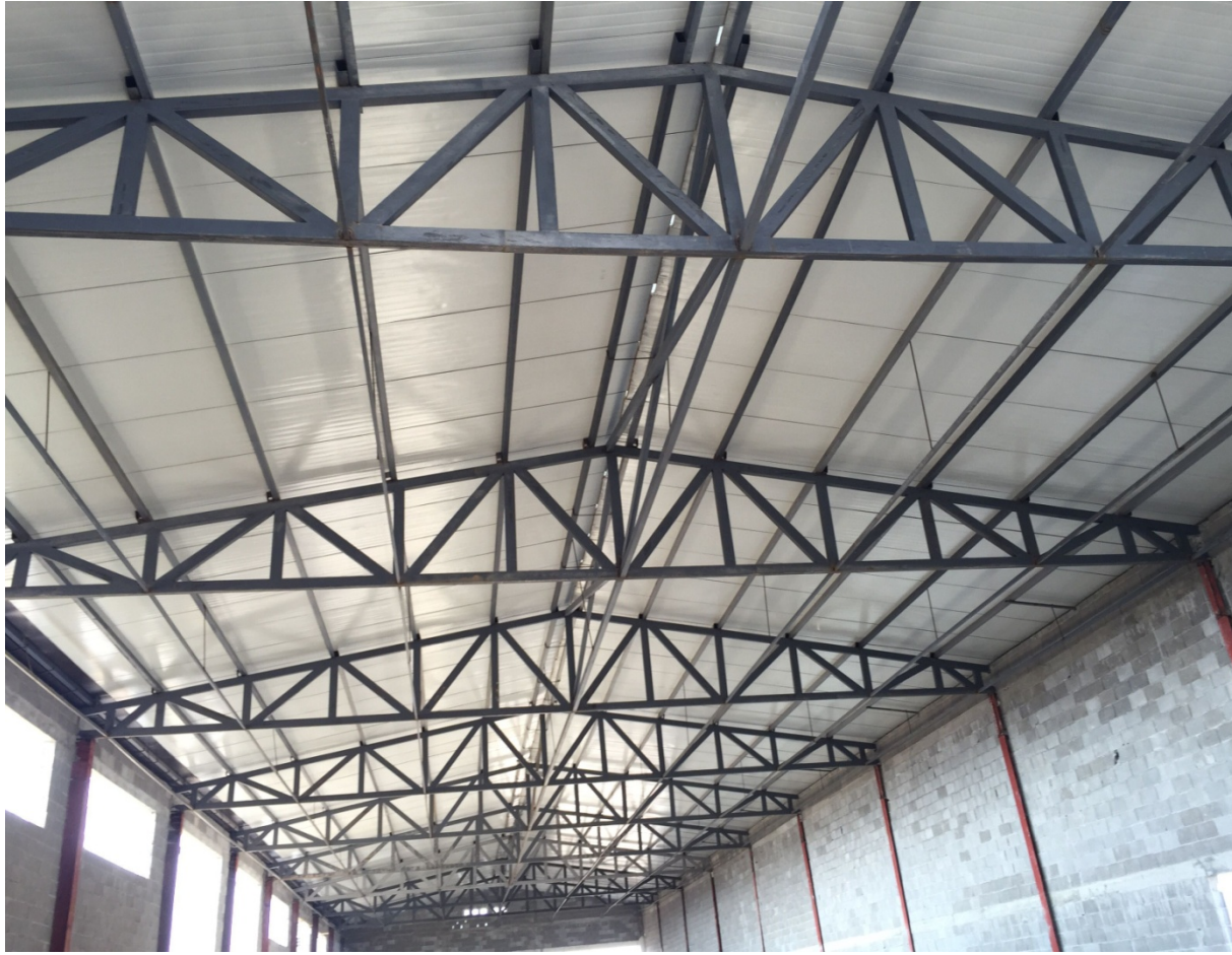
Mbulim I realizuar me panel sandwich(objekti Kosove)
